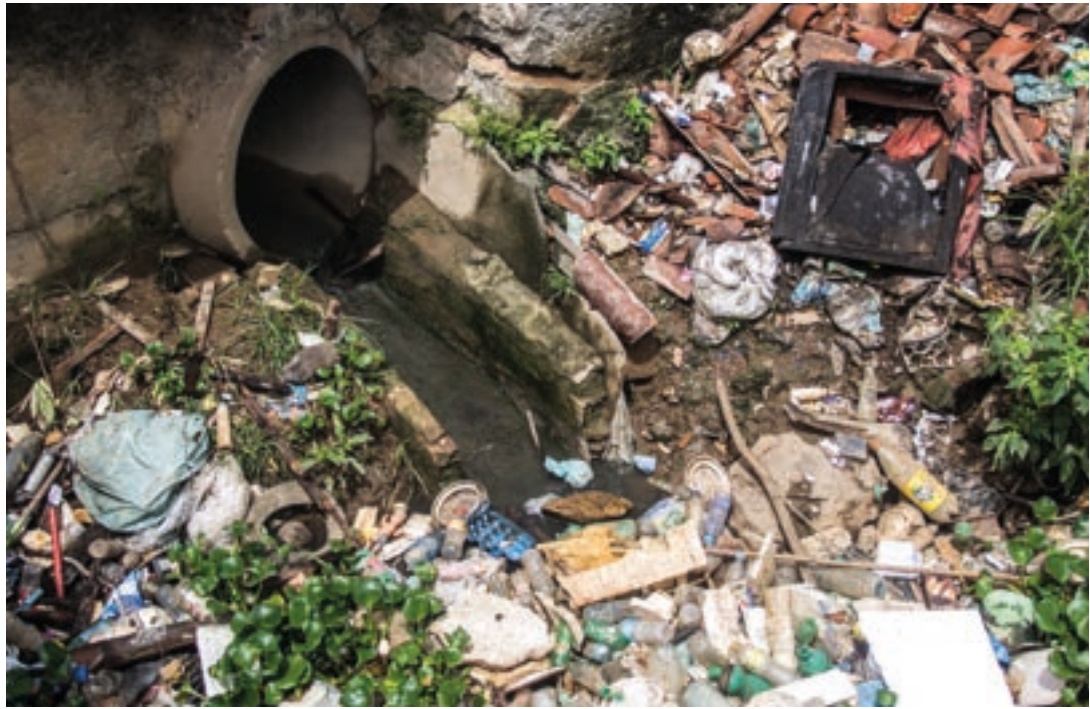
📷 A drainage channel blocked with plastic waste, Brazil. Photo:Moises Lucas Lopes da Silva/Tearfund
